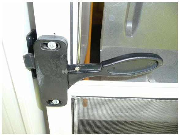
You will have to flex the spoke a little in order to feed the threaded end up through the hole in the plastic door slide stop/handle. The better way to do it is to remove the stop/handle (only two retaining screws) and feed the spoke up through the hole and then replace the handle. This way you don't permanently bend the spoke out of shape.
