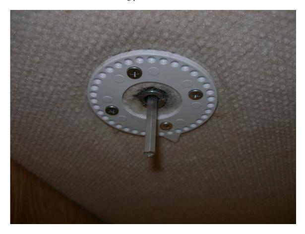
I pre-drilled 3/16" holes thru the Gel-coat and used a 3/32" drill for the plywood beneath and installed (10) #10 X 3/4" Panhead stainless steel screws and washers. I also sealed the base plate with white Dicor (brand) #501-LSW sealant. <a href="http://www.dicor.com/">http://www.dicor.com/</a>
