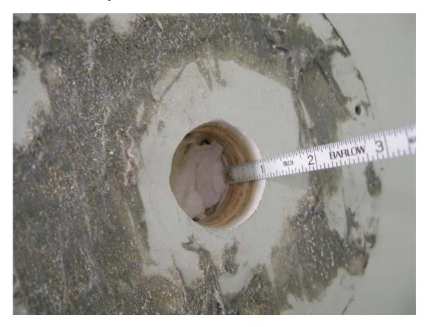
This is a picture of the reverse side of the base plate from the Winegard Sensar III antenna. This is why the hole size needs to be enlarged from  $1\frac{1}{4}$ " to  $1\frac{1}{2}$ ".
