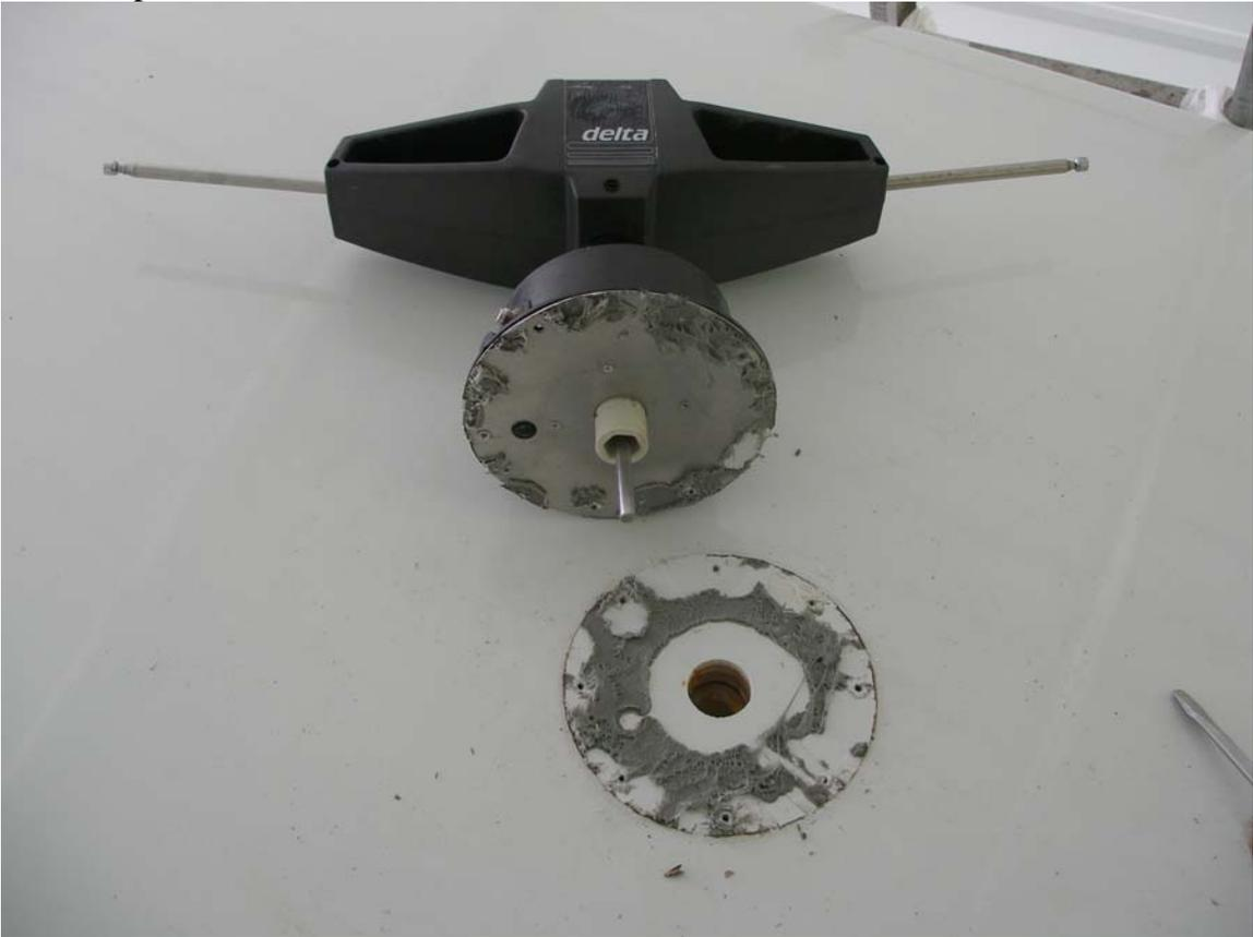
This shows the thickness of the gel-coat (1/4") and the plywood (3/4") the hole is 1 1/4" in diameter. It was very hard to remove this old sealant.
