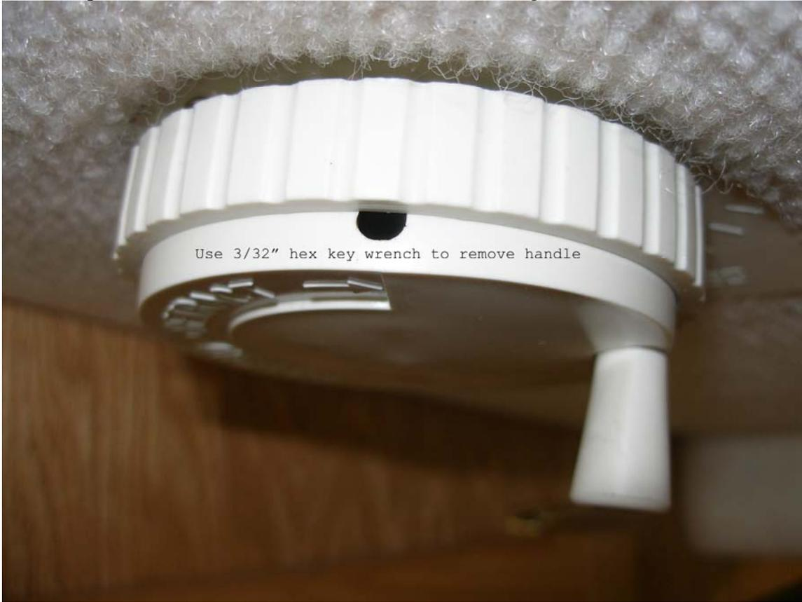
Set screw backed out and handle removed
